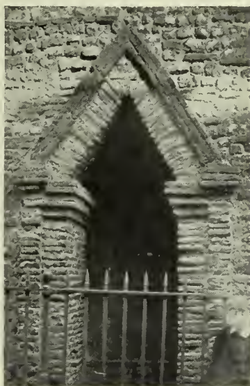
WEST DOORWAY, CHURCH OF HOLY TRINITY, COLCHESTER.
